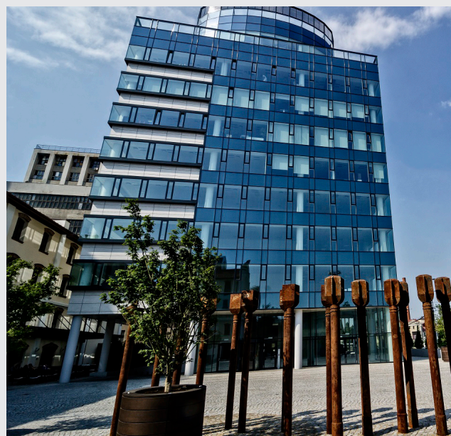
Radisson Collection Belgrade & New Mill Office Building
